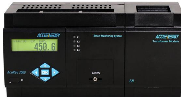
Figure 8: Photo of the Accuenergy AcuREV2000 18-channel meter used for monitoring single-phase circuits in public building environments
